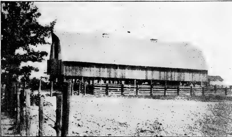
FIG. 12.—Modern cattle barn on the experiment farm at Collins, Miss. With the exception of the roof this barn was constructed of used lumber from abandoned "dummy-line" trestles and mill timbers. Note the storage room above and the daylight underneath.
